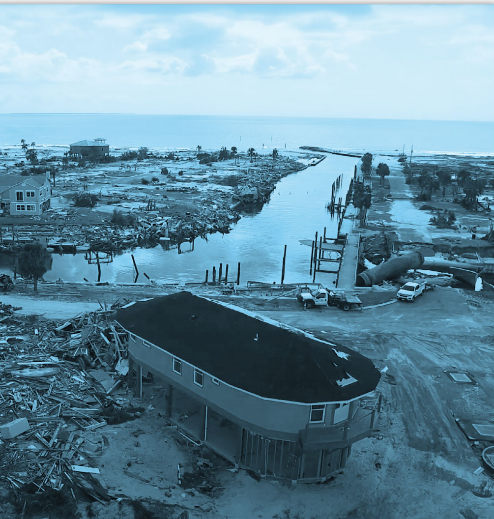
| Deltec home standing after hurricane |
